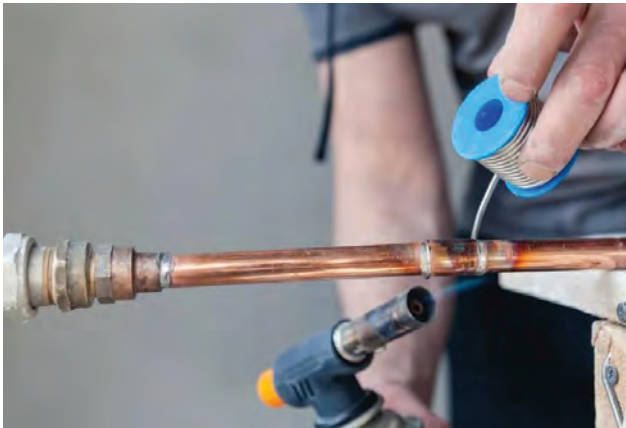
Fig. 1. The process of soldering copper pipes
